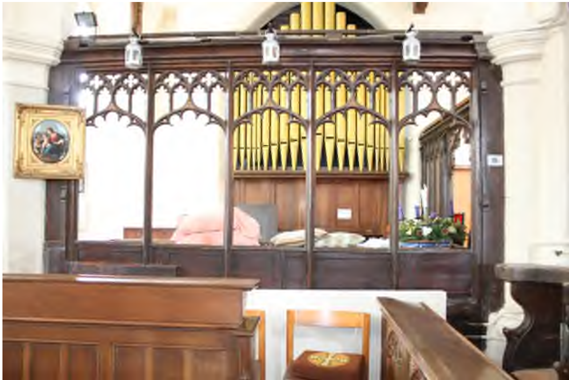
St Nicholas, Stevenage. South face of westerly choir-parclose. Notice mortises in top rail.
